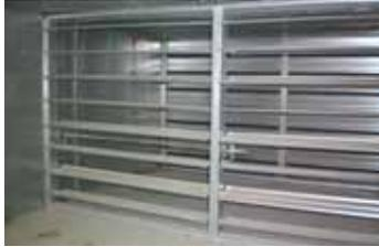
Dampers are supplied with extended shafts shipped loose for field mounting. It is best to drive the dampers from the factory identified driving blade, but in some situations, the preferred blade is not available for driving and another blade is required.
