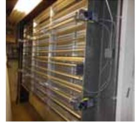
Spring return actuators are also known as fail-safe actuators because they return the damper to an open or closed position that is safe for the environment where the damper is located.
