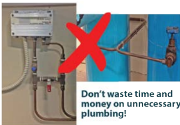
Remote sensors eliminate need for bypasses
