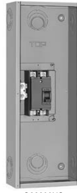
Q22200NS With Cover Removed
