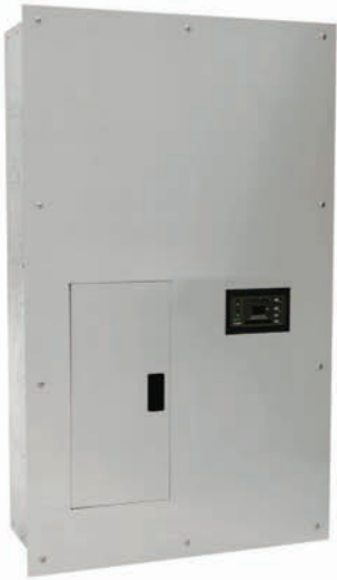
Operating Room Isolated Power Panel
