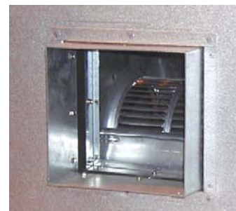
Flex collar at discharge
