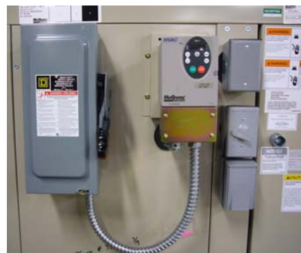
Disconnect, starter and vfd
